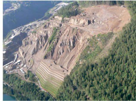
Figure 7. Aerophotogram of the reinforced steep slope completed.
