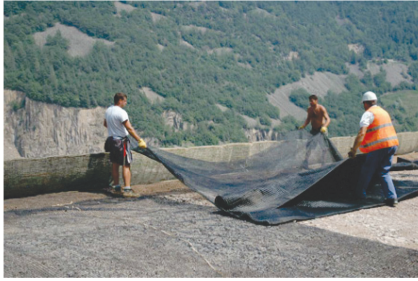
Figure 5. Installation of primary reinforcing geogrid.
