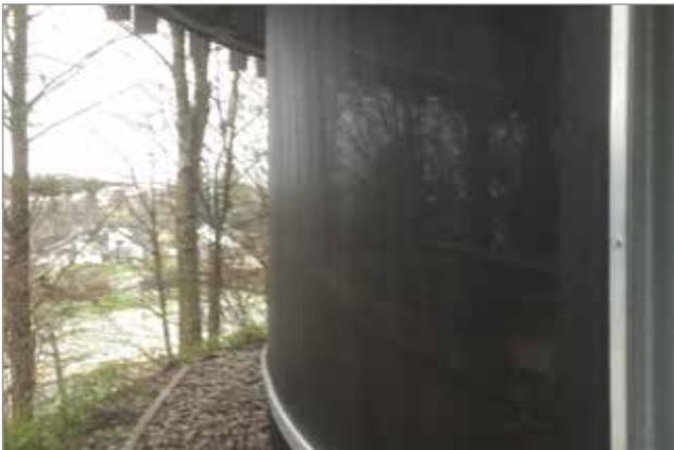
Curved section, installed with rolled aluminium keder rails
