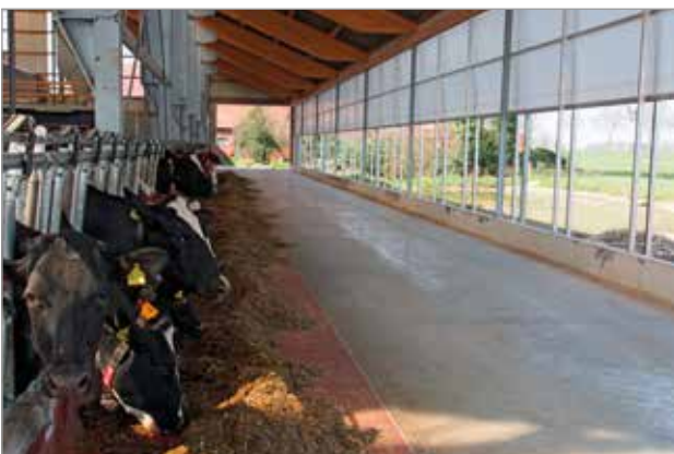
Interior view of Lubratec WLU-XL „bottom opening – central roller“ roll-up ventilation
