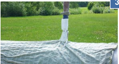
Concreting via filler neck
