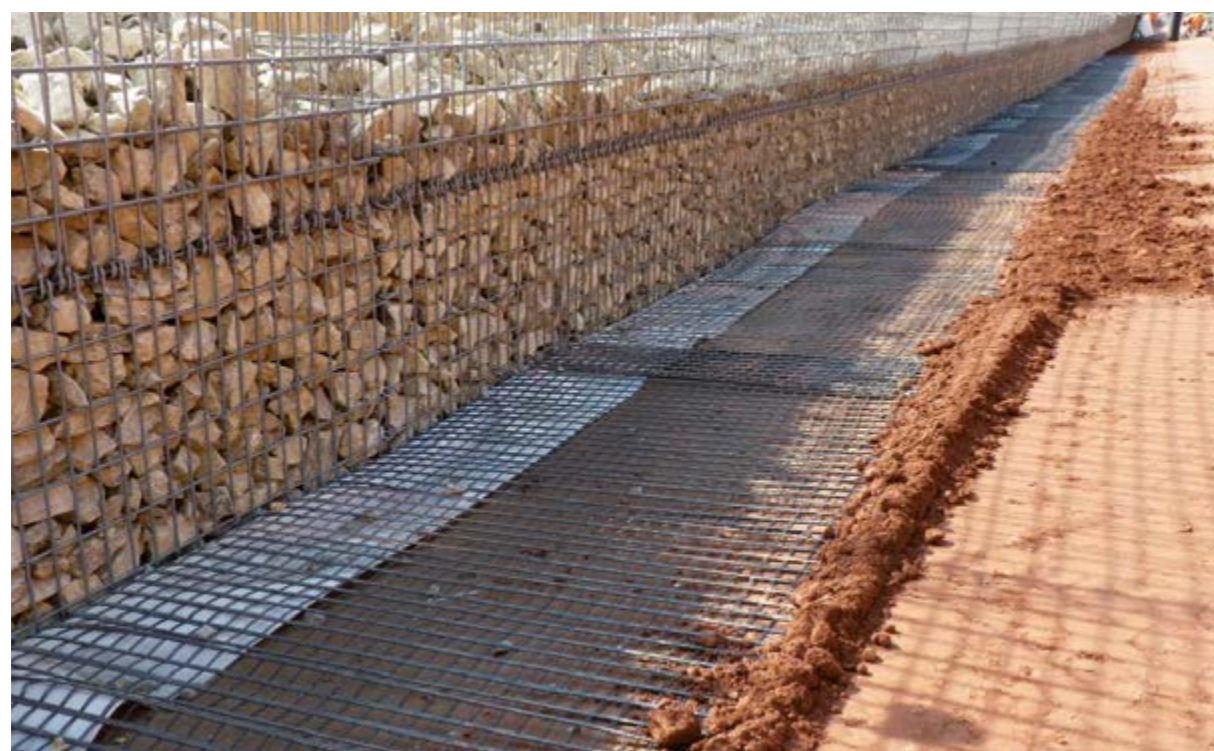
Tied-back gabion wall (A3 motorway near Haseltal, Germany)
