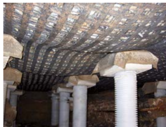
Membrane effect in piled embankment application (Railway Bidor-Rawang, Malaysia)
