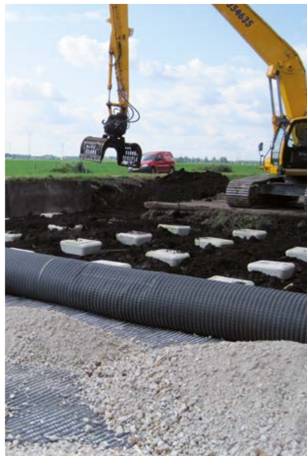
Geotextile reinforcement installed on piles (N 210; Netherlands)
