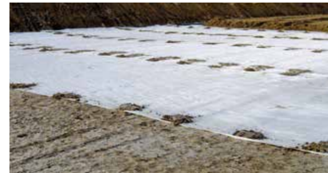
Ballasted /overlapping sheets
