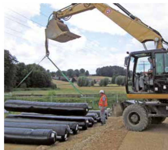
Use of lifting /laying gear
