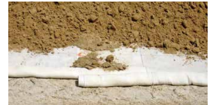
Overlapping sheets with soil cover
