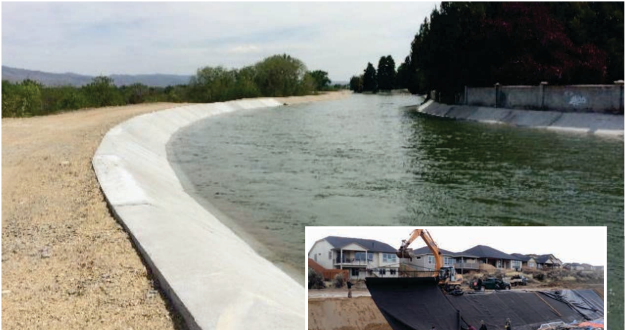
Completed lined canal section
