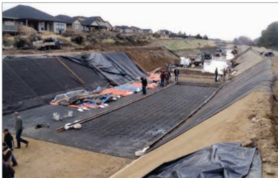
Installation of concrete screed and #4 rebar for placement of 6-inch concrete
