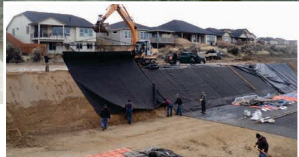
Installation of Canal3 123012 by Boise Project Board of Control personnel
