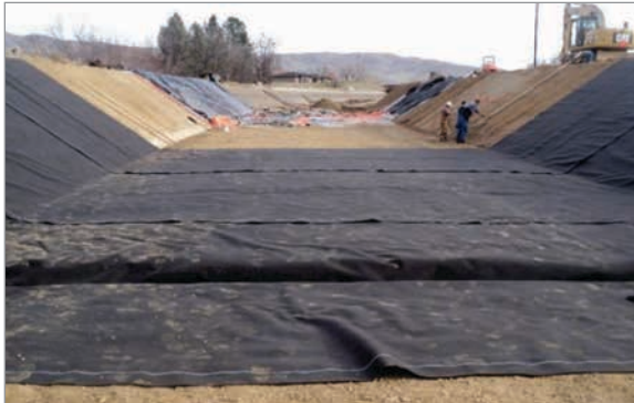
Anchor trench across end of canal section for future installation
