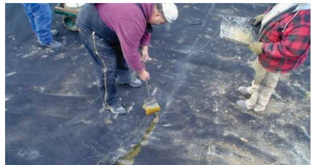
Seaming Canal 3 123012 using hot melt adhesive
