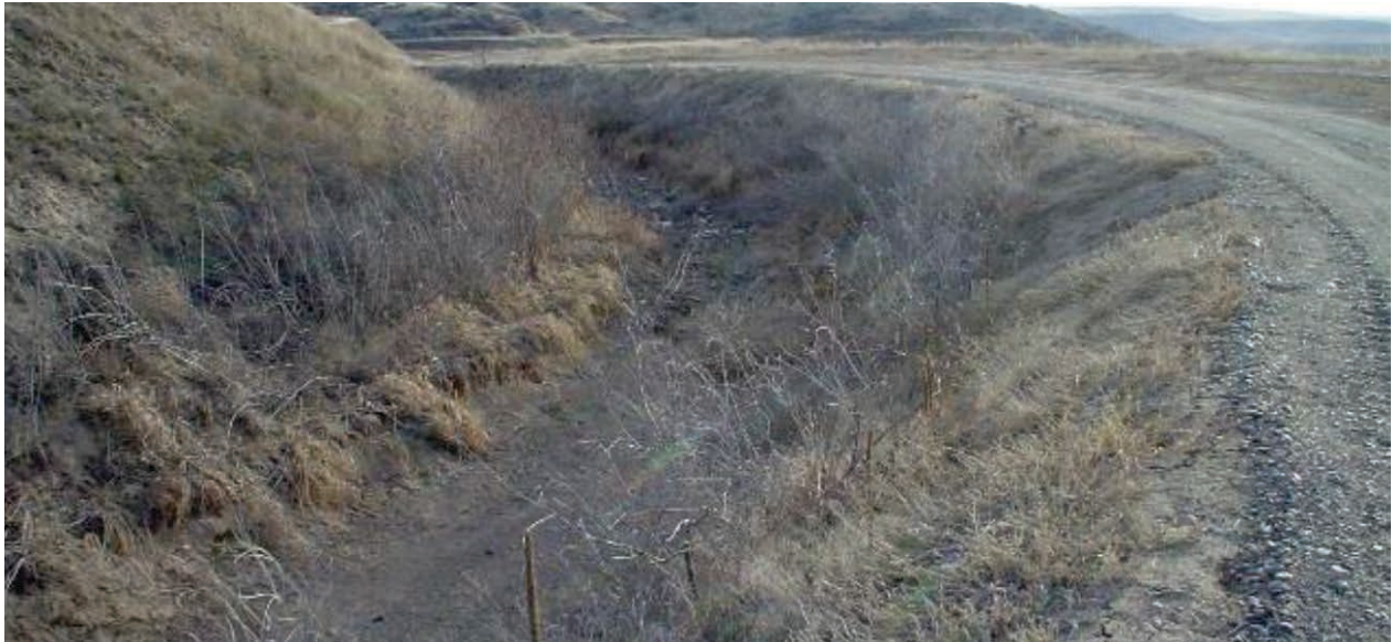
Unlined irrigation canal
