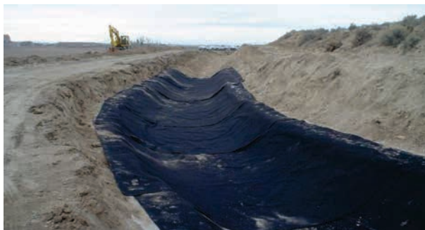
Canal 3 123012 installed perpendicular to the canal
