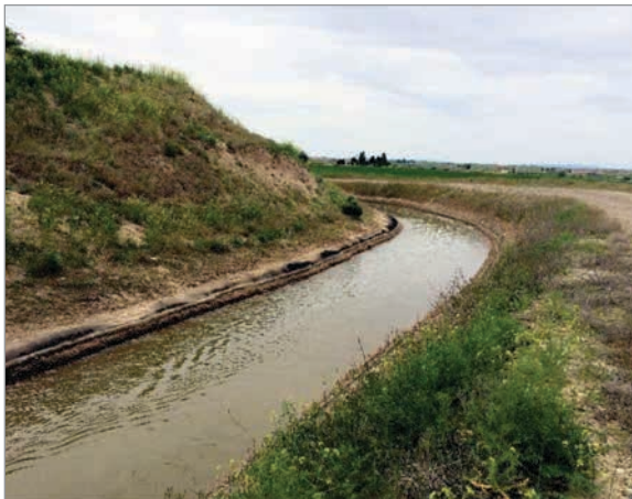
Completed exposed lined canal
