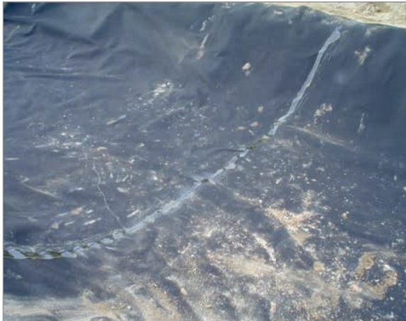
Completed seamed section
