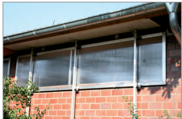
Lift window seen from outside
