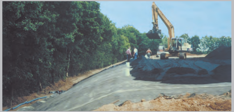
Landfill capping with NaBento®
