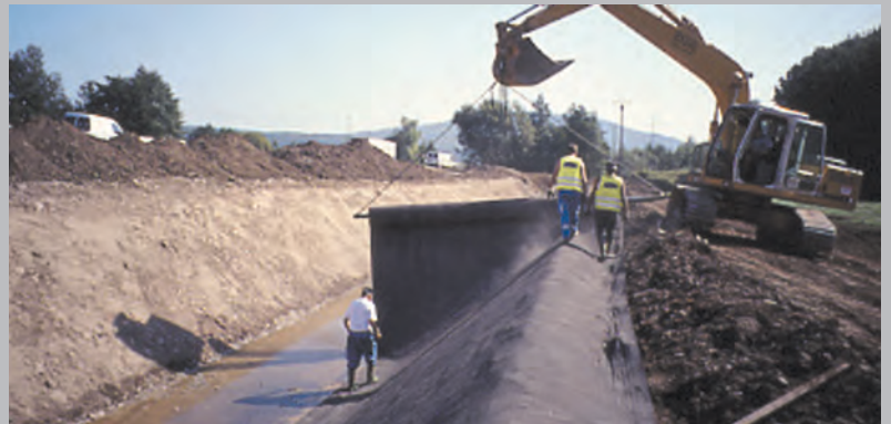
River-bed lining with NaBento®
