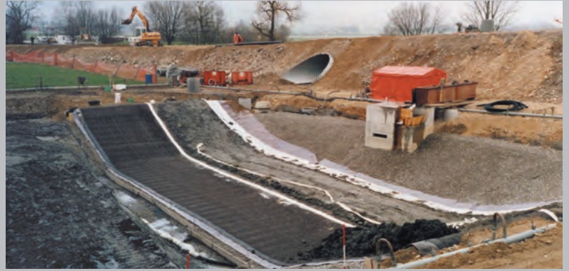
Settlement lagoons - Lining with NaBento®
