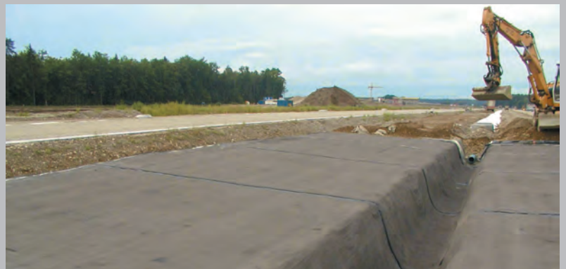
Groundwater protection on a road scheme
