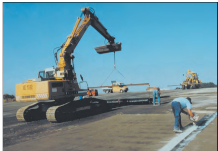
NaBento®- installation in a landfill construction
