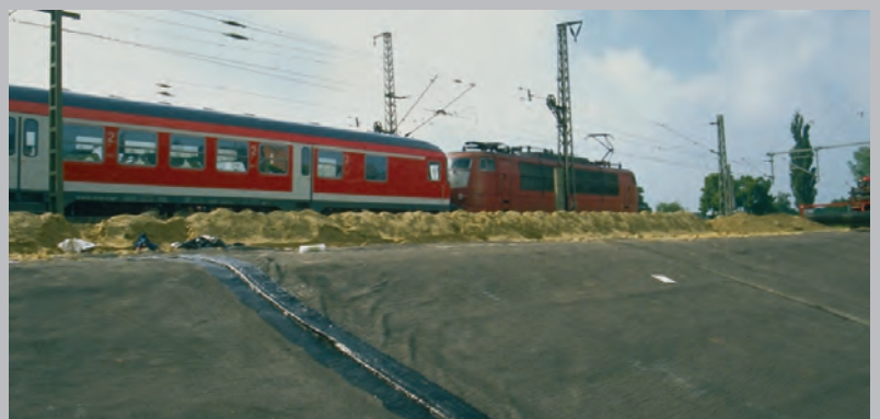
Railway lining with NaBento®
