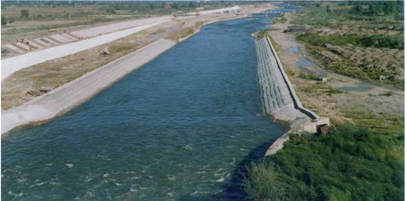
Slope protection with Incomat® Flex
