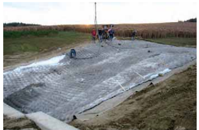
Incomat® FP after filling with concrete (2)
