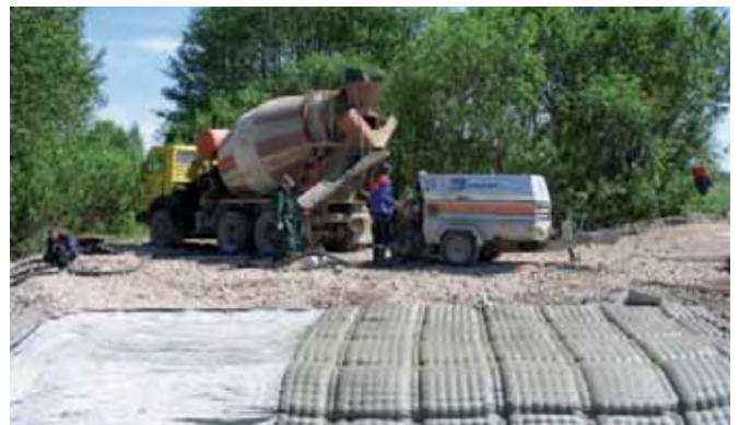
Installation of Incomat® Flex
