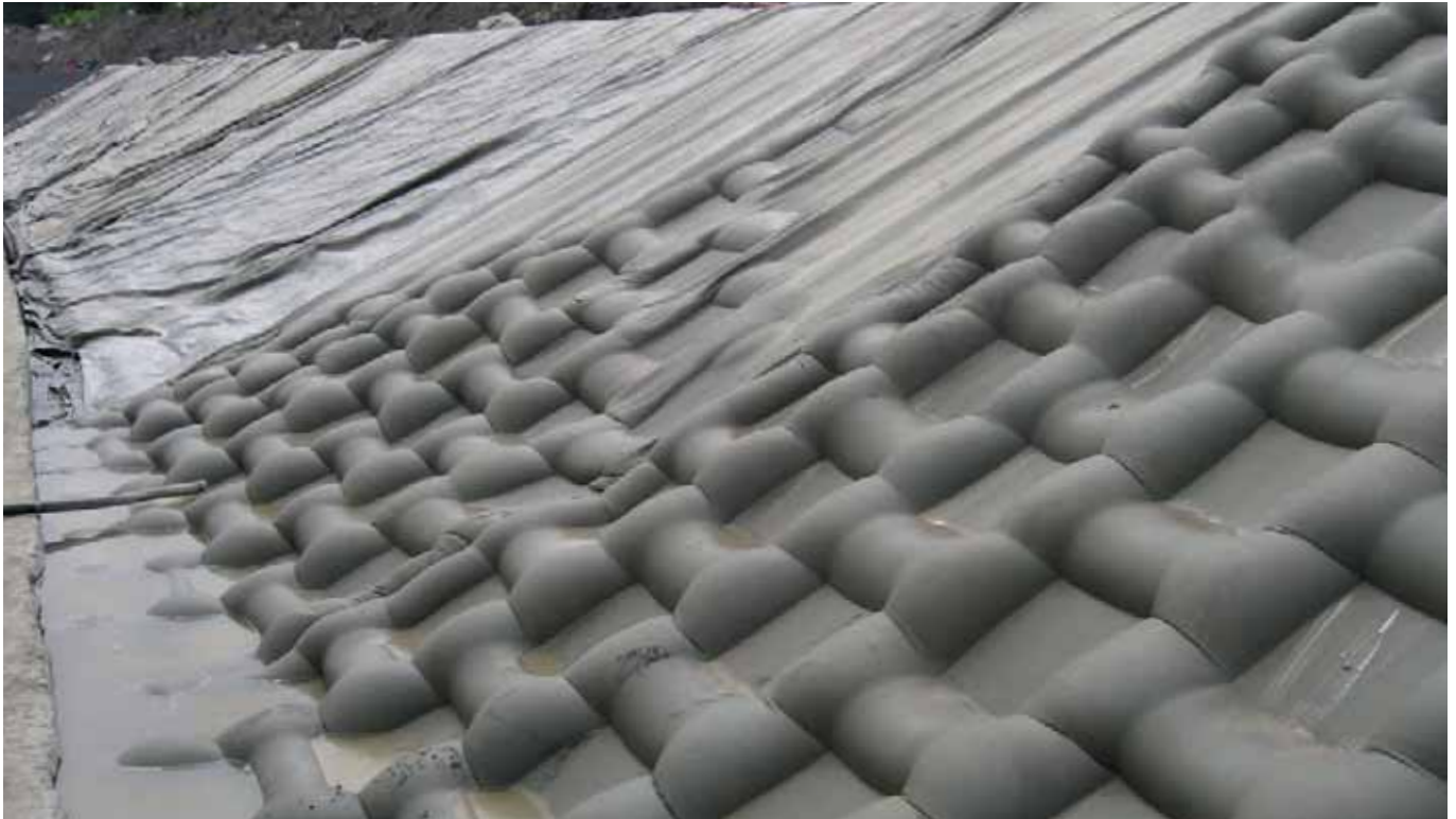
Installation of Incomat® Crib
