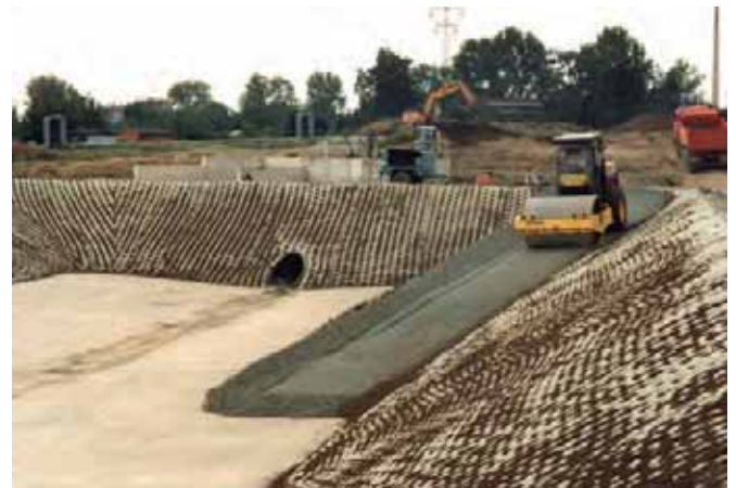
Attenuation pond with Incomat® Crib after apertures have been filled with soil (2)
