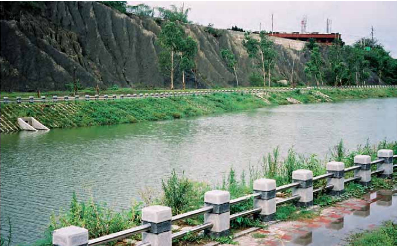
Established vegetation after construction (3)
