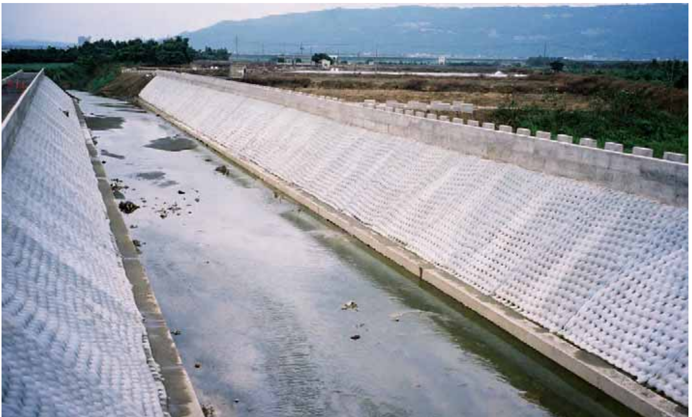
Completed canal lining using Incomat® FP
