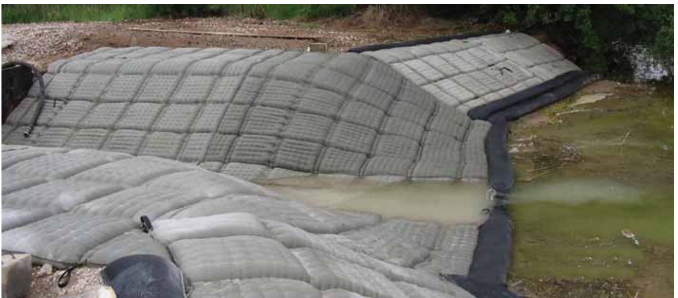
Repaired outlet after completion (4)
