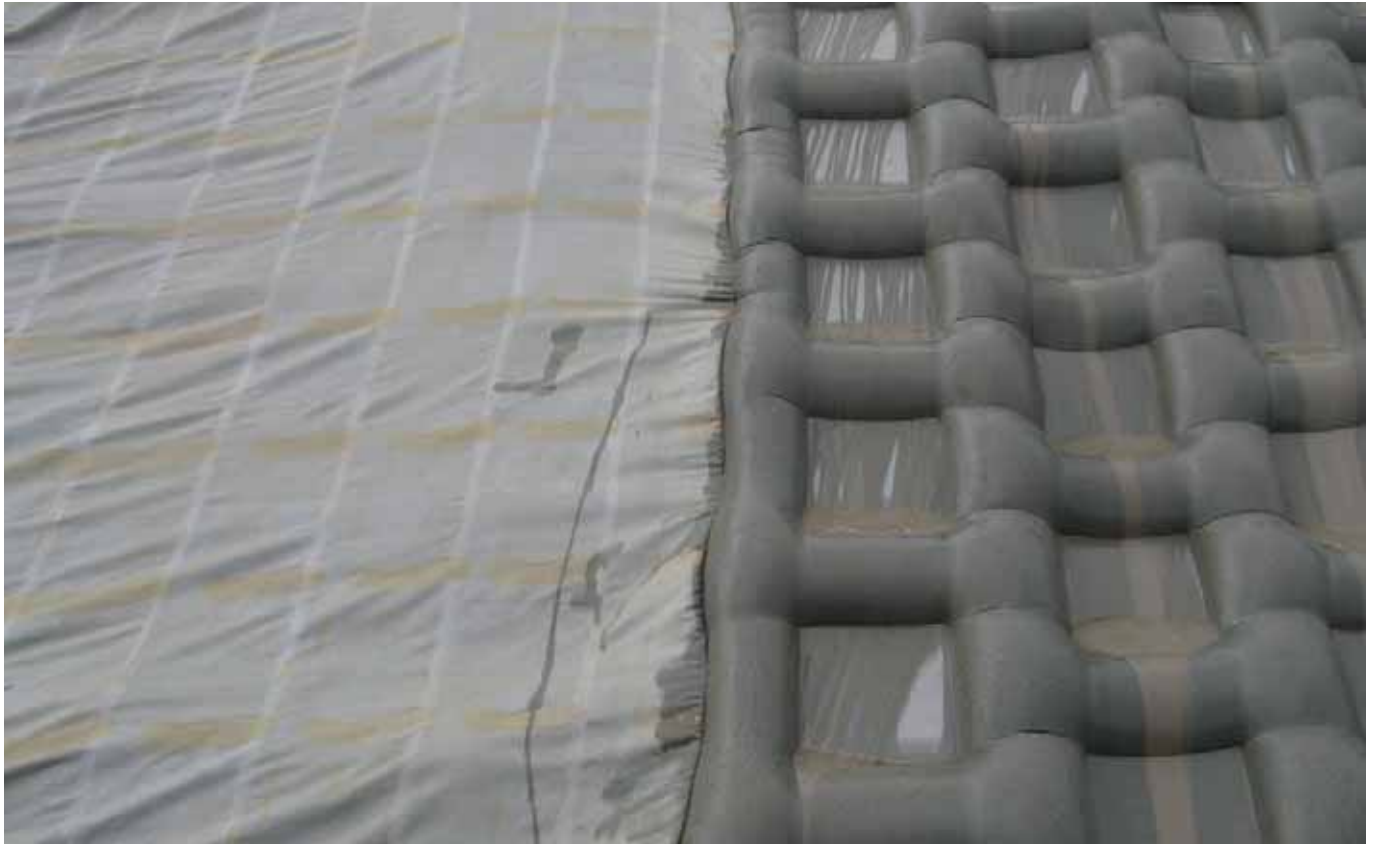
Sewn connection between two Incomat® Crib panels (left unfilled – right filled)
