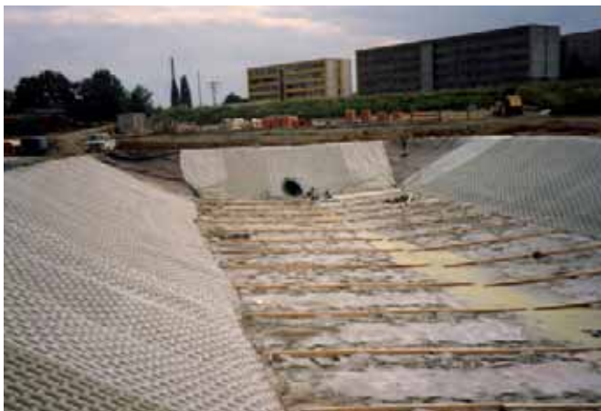
Attenuation pond with Incomat® Crib during construction (1)
