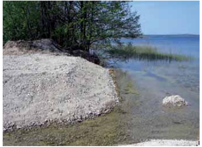
Slope preparation (earth works) (2)
