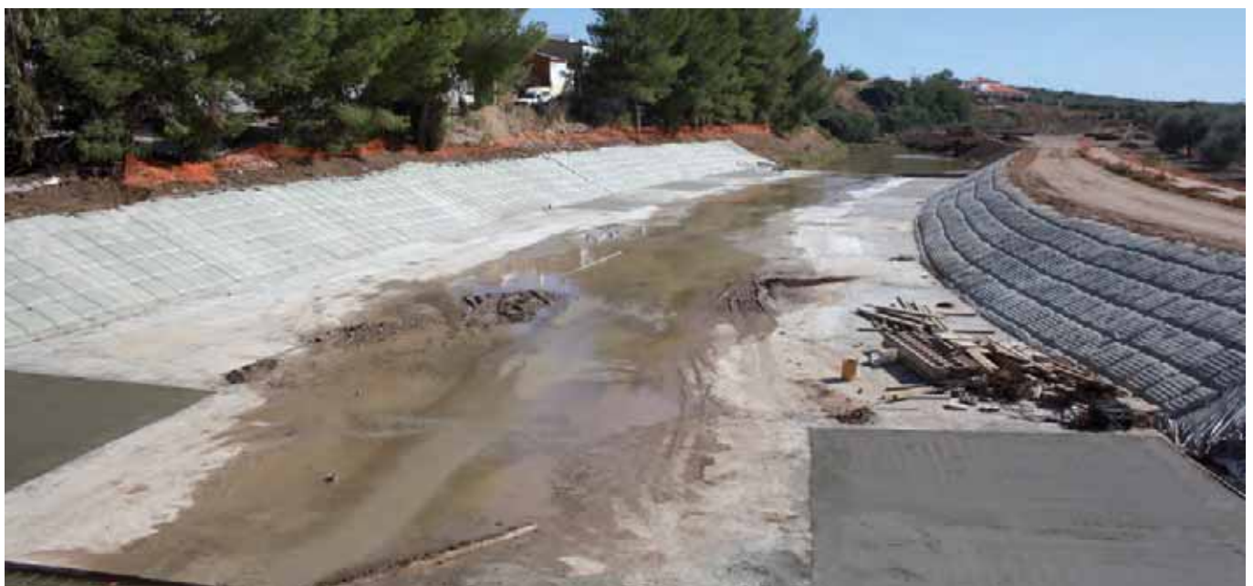
Slope protection with Incomat® Flex
