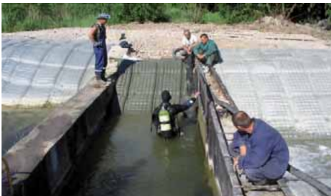
Installation of Incomat® Flex under water
