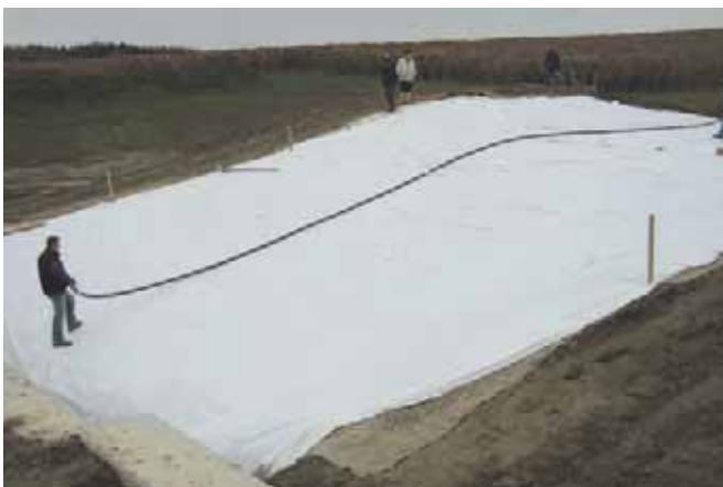
Incomat® FP prepared for installation (1)
