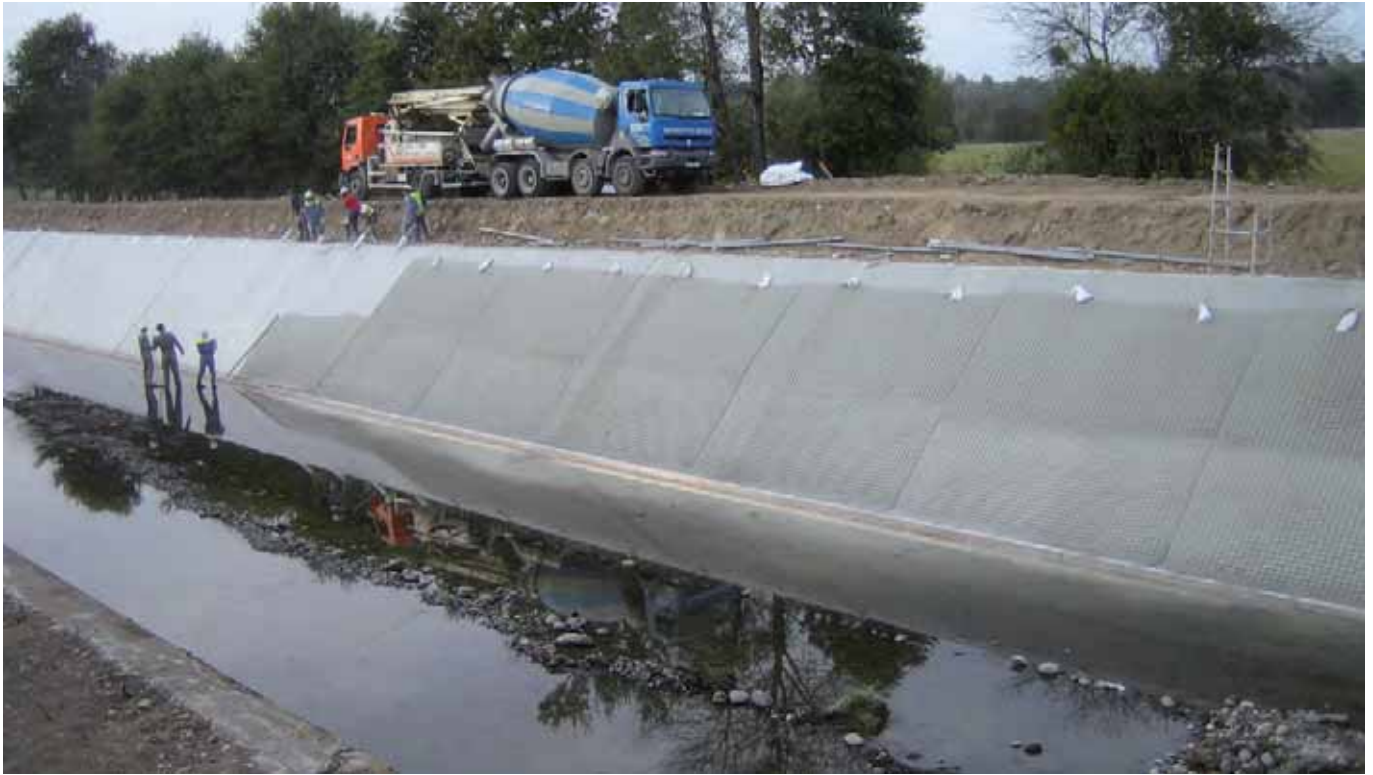
Progressive filling process of Incomat®
