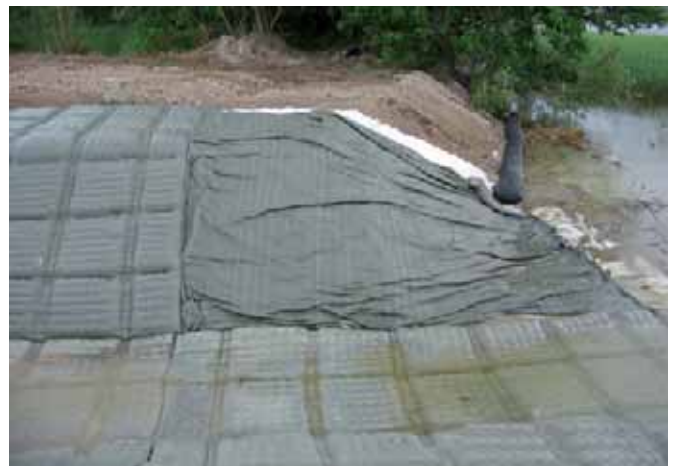
Installation (filled and unfilled section) (3)
