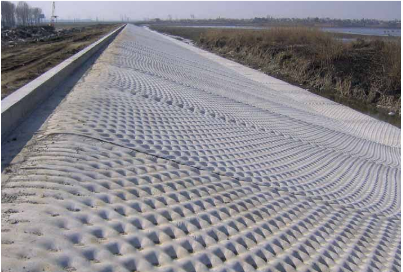
Slope protection with Incomat® FP
