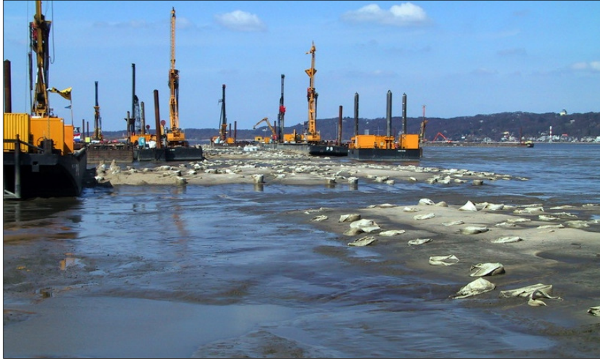
Figure 1. Installation of GECs (Ringtrac) over water and extremely soft mud
