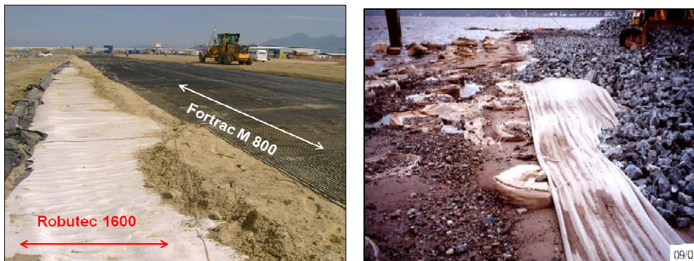
Figure 6. Example of horizontal geosynthetic reinforcement on top of already covered GECs for heavy loaded sensitive runways (left) and under a land reclamation embankment (GECs still visible) (right)
