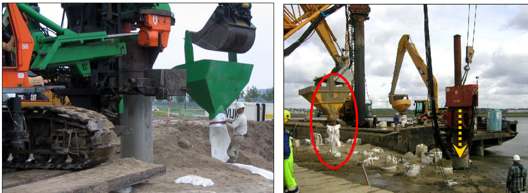
Figure 8. Installation of geotextile encasement
