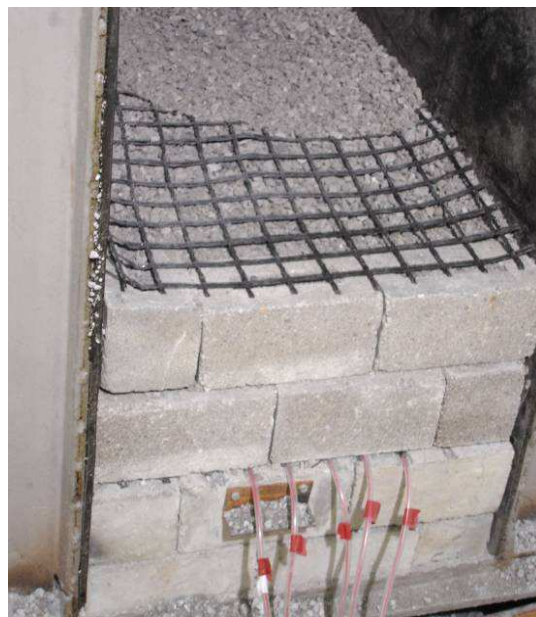
Fig. 3. Installation of geogrids with frictional connection to the facing blocks
