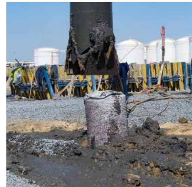
Ground improvement for oil tanks Spain: construction of safe, ductile foundation system in very soft soils with Ringtrac geotextile-encased columns.
