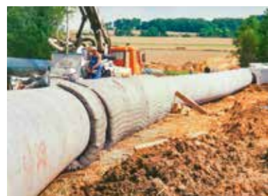
1997 Pipe encasement, inverted siphon, France, River Luce, gas pipeline
