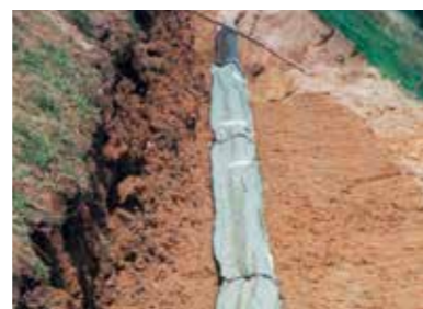
2006 Pipe cover, France, gas pipeline
