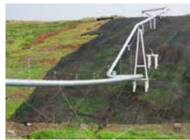
2004 Slope stabilization, Russia, Baku-Novorossiysk, oil pipeline
