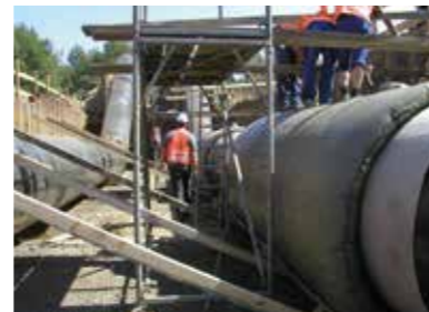
2009 Pipe encasement, inverted siphon, Germany, Essen, gas pipeline
