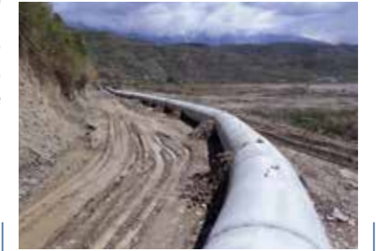
2017 Pipe encasement, Greece and Albania, TAP, gas pipeline
