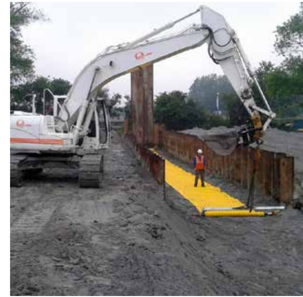
Artère des Hauts de France, DN 900 France: early warning system and excavation protection for gas pipeline with Fortrac PipeGuard geogrid.
