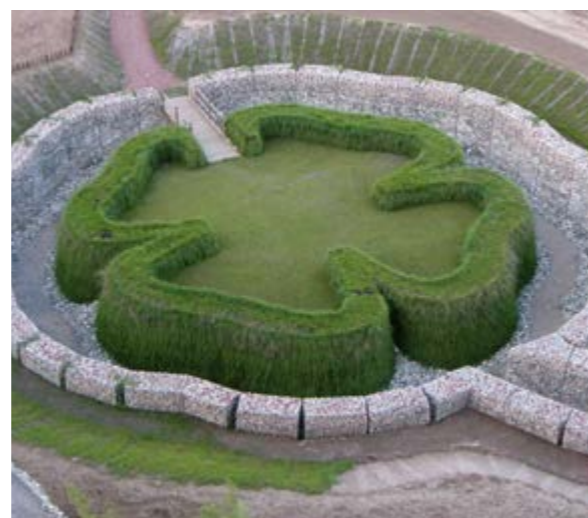
Trèfle art installation in Parco Arte Vivente, Turin Italy | Permanent landscape artwork shaped like a four-leaf clover – Fanciful architectural concept made possible by Fortrac geogrid’s high flexibility – System with integrated lost formwork.
