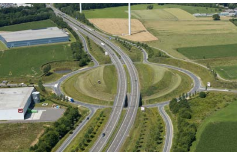
Buitenring Parkstad Limburg megaproject Netherlands | 26 km bypass with links to A76 motorway and N281 urban motorway– Total 39 structures (e.g. ramps, steep slopes, noise barriers) includes 30 bridge abutments – In all, some 650,000 m² Fortrac geogrids incorporated.
