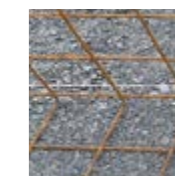
Lost or temporary formwork for passive facing
