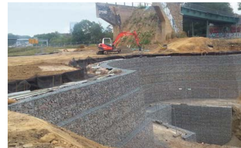
Uncovering of River Schondelle Germany | Sub-project of River Emscher ecological improvement scheme – Earthworks built with integrated lost formwork and full-gabion facing – Solution as replacement for originally planned concrete cantilever wall – Erected in three, 5 m tall vertical sections.
