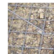
Galvanised steel formwork units
