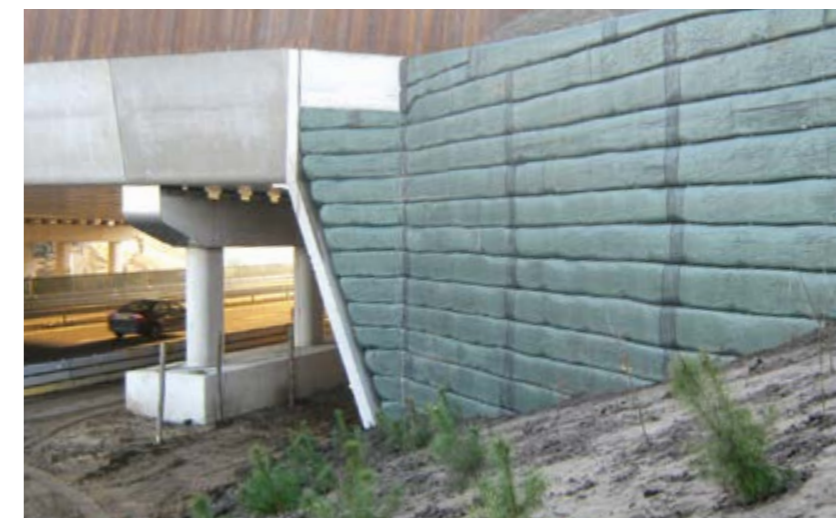
The first 110° earth pressure relief wall in the world Netherlands | Vegetated wildlife bridge over A2 motorway with 110° earth pressure relief wall – Only cost-efficient option available to shield slender concrete structure from earth pressure – Adopted solution also incorporates steel mesh facing and vegetation.
