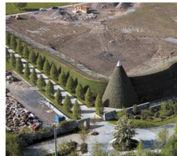
New residential estate near motorway, Iserlohn Germany | Terrain raised by up to 25 m to create residential site – Combination of 90° retaining wall and 80° noise bund – High soil pH values – Alkali-resistant Fortrac (PVA) geogrids specified – System with integrated lost formwork – Instrumentation installed for long-term monitoring.
