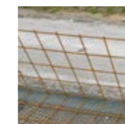
Ungalvanised steel formwork units
