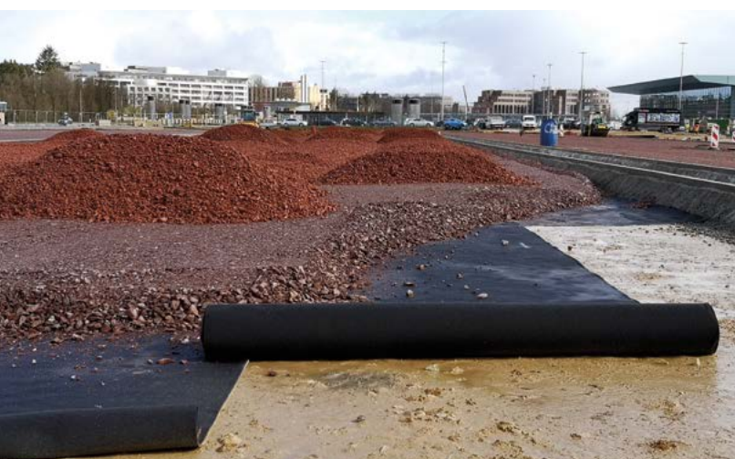
Pollutant filter under parking lot Luxembourg | Tektoseal Active AS was laid underneath the gravel layer of a parking lot to prevent contaminants from entering the subsoil. Tektoseal Active AS allows water to pass through and has been proven to reliably absorb oils and fuels as well as pollutants such as metals that stick to particles. This allows for the safe design of water-permeable traffic areas.
