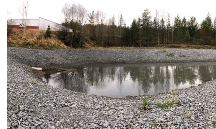
Mine water treatment Finland | Mine drainage containing metal can also be treated in basins next to pits and heaps. For mine water treatment in a closed nickel mine, two filter basins were lined with Tektoseal Active HM.
