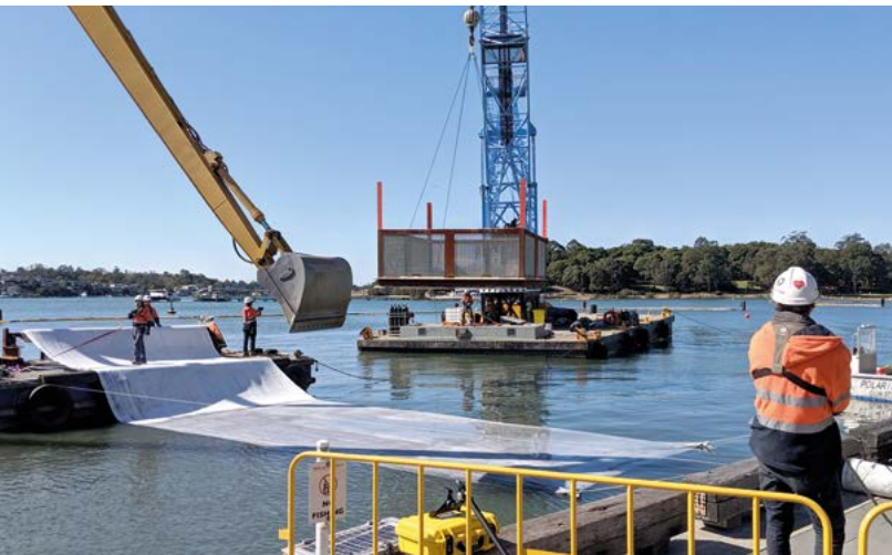
Securing of contaminated sediments Australia | Securing sediments with high PAH and CHC contamination in a Sydney bay. Installation of approx. 5,000 m 2 of Tektoseal Active AC as a pollutant barrier layer for improving the water quality.
