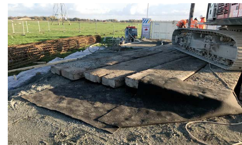
Working in groundwater protection zones Germany | Construction work in groundwater protection zones requires special attention to soil and water protection. Leaking lubricants and fuels from construction machinery are a hazard that is contained by Tektoseal Active AS. In this project, the contaminant filter was used under a large rotary drilling rig.
