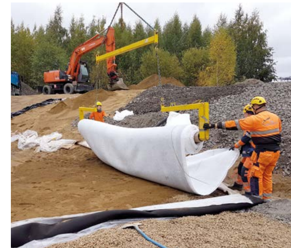
Surface runoff treatment Finland | Surface runoff from sealed areas contaminated with PAH and CHC is treated in a stormwater retention basin. By installing Tektoseal Active AS and AC in the bottom of the pond, pollutants are filtered out of the water before it seeps away. The basin walls are largely impermeable to water and lined with a geosynthetic clay liner.
