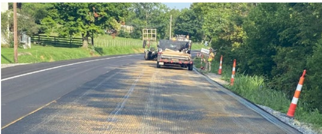
Sanding HaTelit to prevent "bleed-through"
