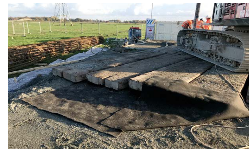
Working in groundwater protection zones Germany | Construction work in groundwater protection zones requires special attention to soil and water protection. Leaking lubricants and fuels from construction machinery are a hazard that is contained by Tektoseal Active AS. In this project, the contaminant filter was used under a large rotary drilling rig.
