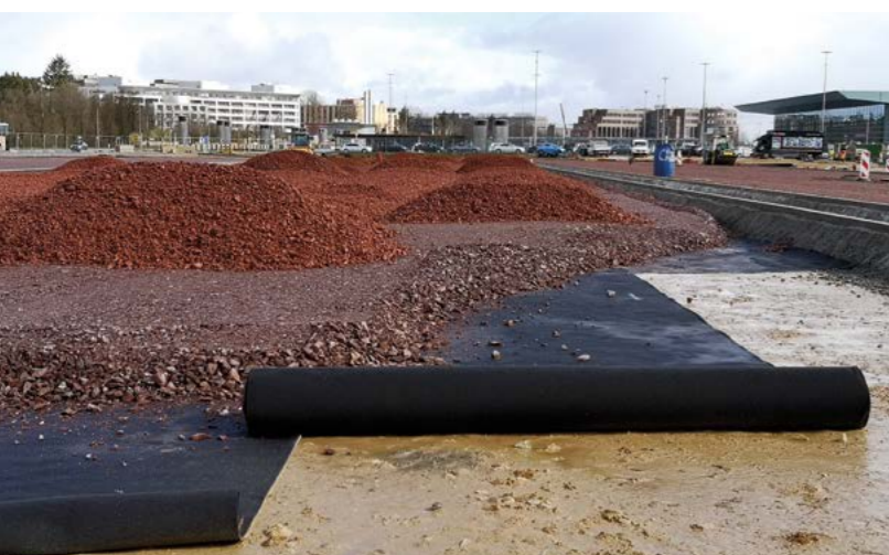
Pollutant filter under parking lot Luxembourg | Tektoseal Active AS was laid underneath the gravel layer of a parking lot to prevent contaminants from entering the subsoil. Tektoseal Active AS allows water to pass through and has been proven to reliably absorb oils and fuels as well as pollutants such as metals that stick to particles. This allows for the safe design of water-permeable traffic areas.
